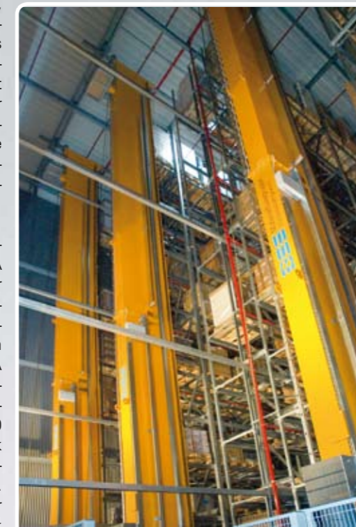
Hochregallager High-bay warehouse
