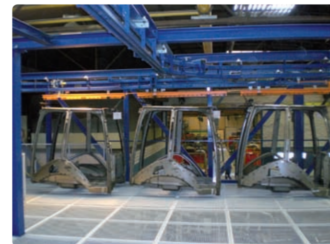
Pufferstrecke: Abgabehuber an Lackierlinie Buffer area: discharge station to paint line
